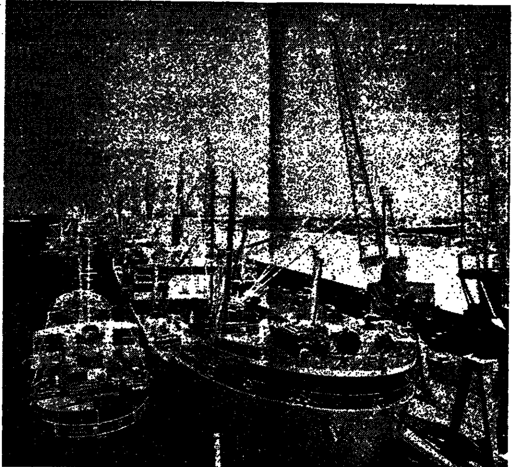
General cargo berths at Jeddah, Saudi Arabia. The port is currently being extended under a scheme which will more than double its capacity. Consulting engineers are Sir William Halcrow and Partners.
